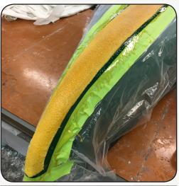
8. Brush firmly and evenly, feathering the edges of the felt to get a level surface. Once the resin has gelled enough to not run (roughly 15 minutes), remove the drip cover and tape outline. Feel free to smooth the edges of the resin-surface with a gloved finger or wedge for uniform adhesion.
